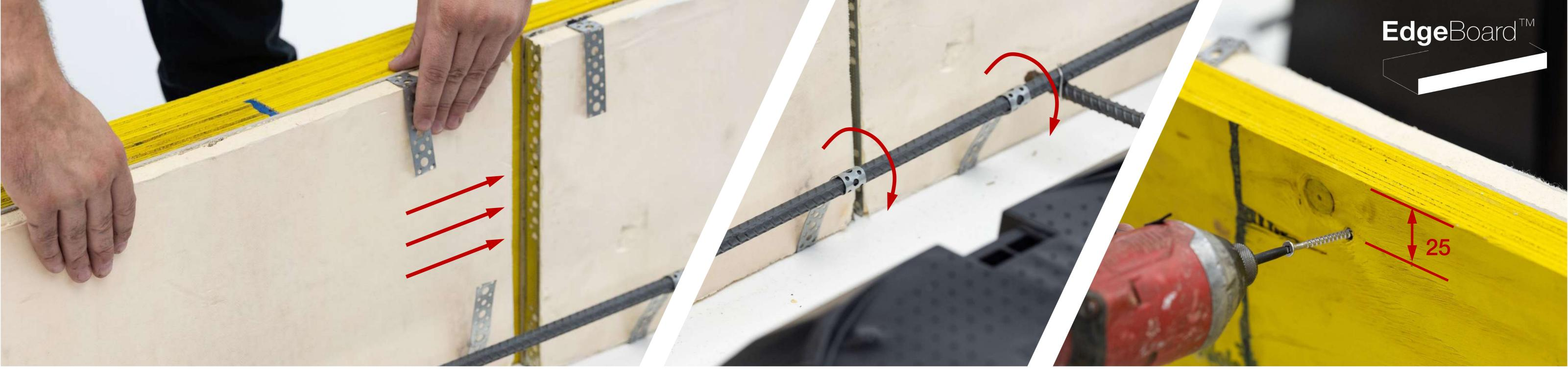
1. Before you start, make sure that the board corner bead is clean and dry. Remove the liner of the double-sided adhesive tape, position and apply some pressure when you connect the boards together.
