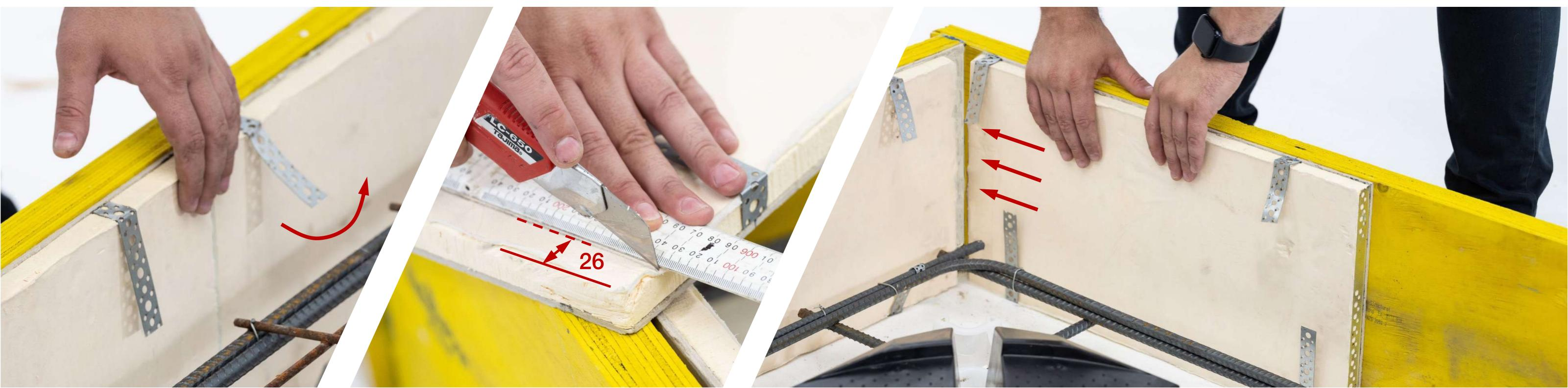
2. Secure the boards by folding the lower clips around the reinforcing bars of the foundation.
