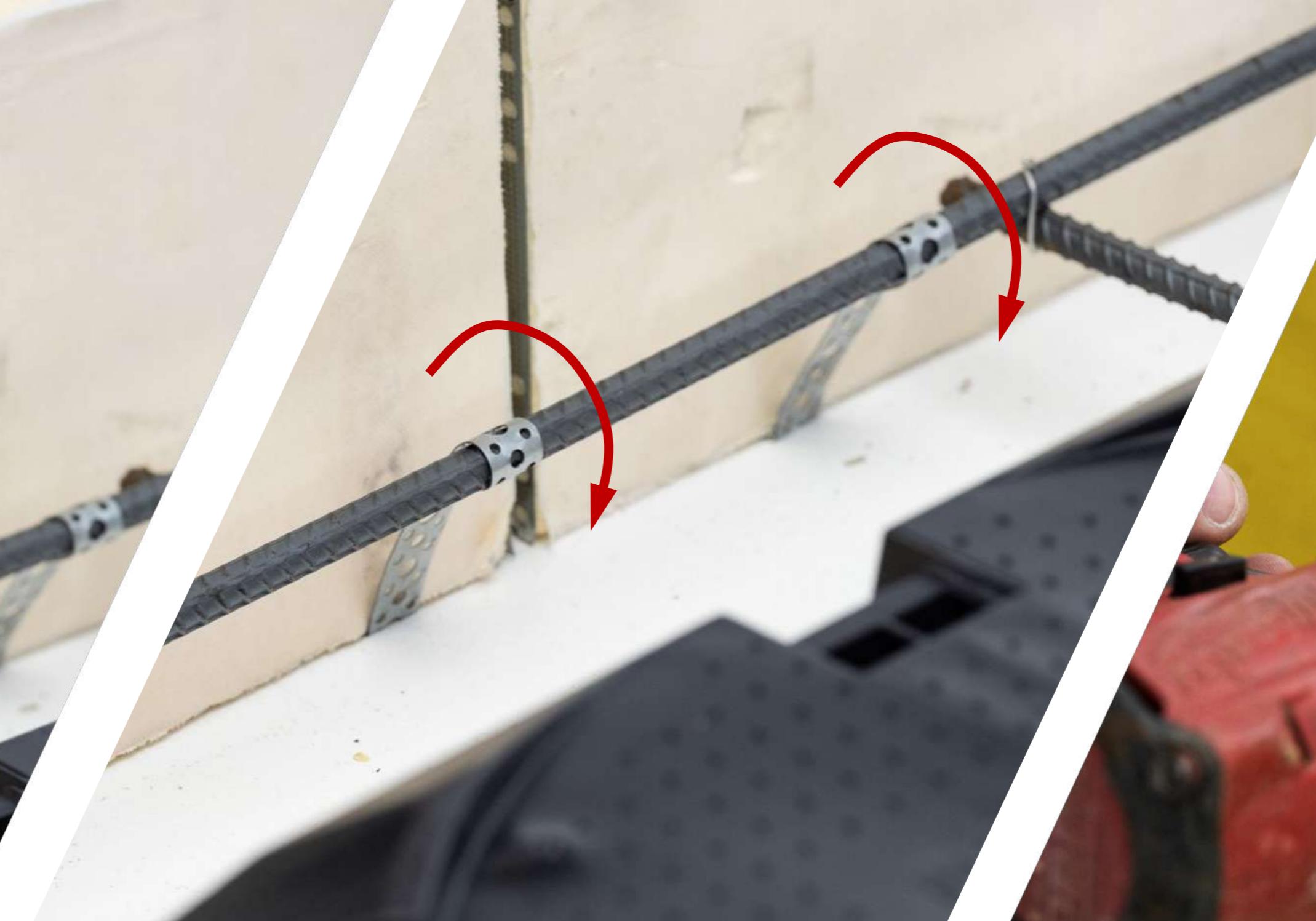
2. Secure the boards by folding the lower clips around the reinforcing bars of the foundation.
