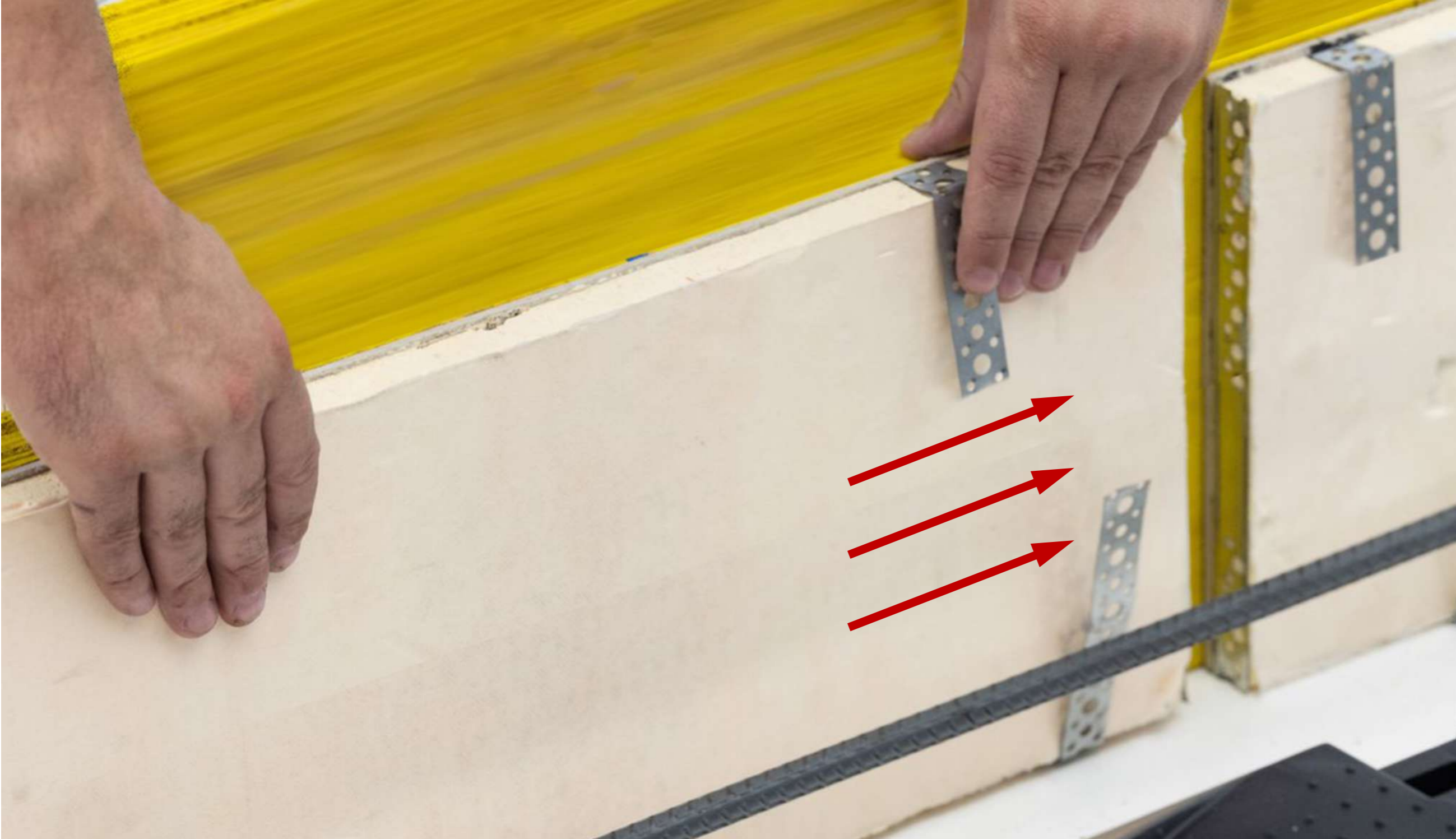
1. Before you start, make sure that the board corner bead is clean and dry. Remove the liner of the double-sided adhesive tape, position and apply some pressure when you connect the boards together.
