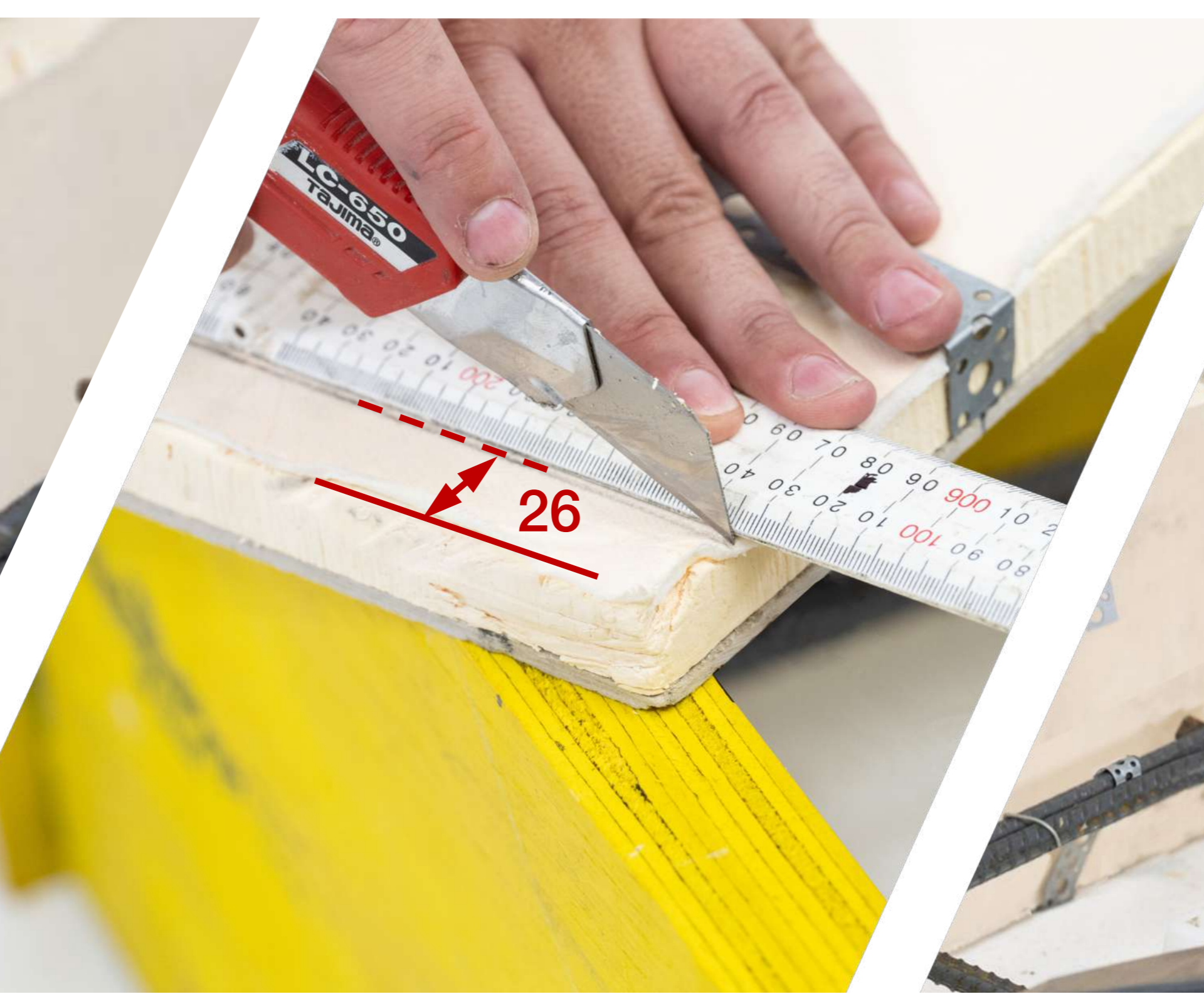
5. At outer corners, cut off a strip of insulation layer. (No cuts are required at inner corners).
