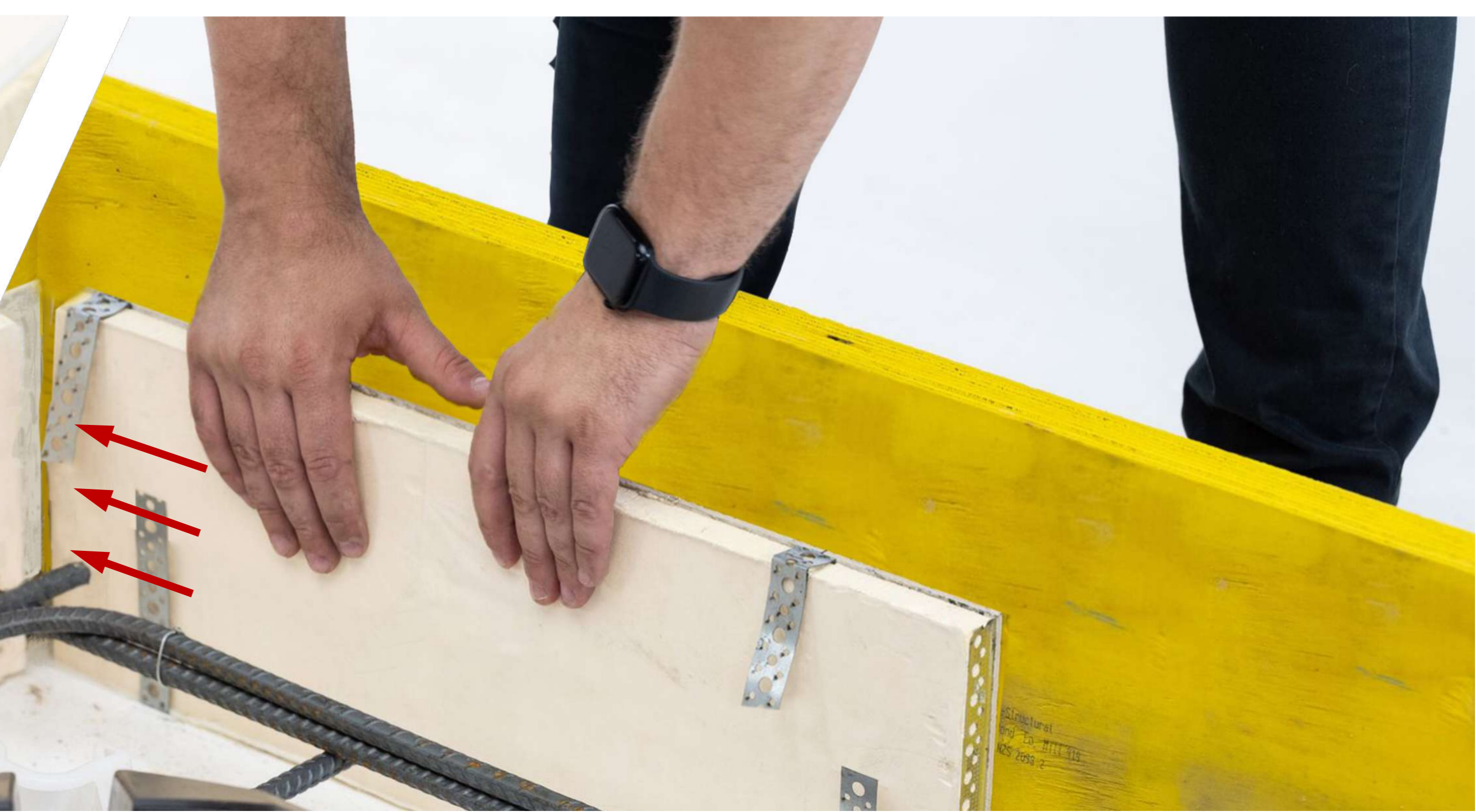
6. Position and connect the boards together. At foundation corners, we recommend fixing each end of the boards to the boxing with self-tapping screws (see point 3).
