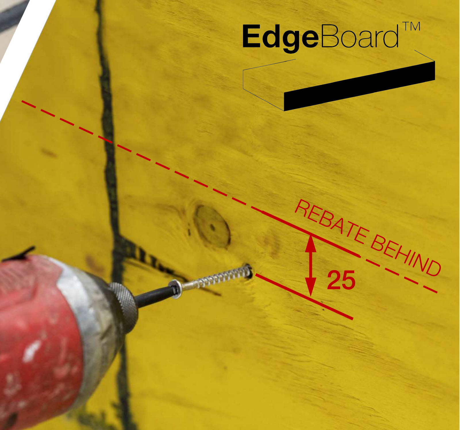
3. For superior stability during construction, temporary fix the board to the boxing along the length with self-tapping screws (1 screw every meter).
